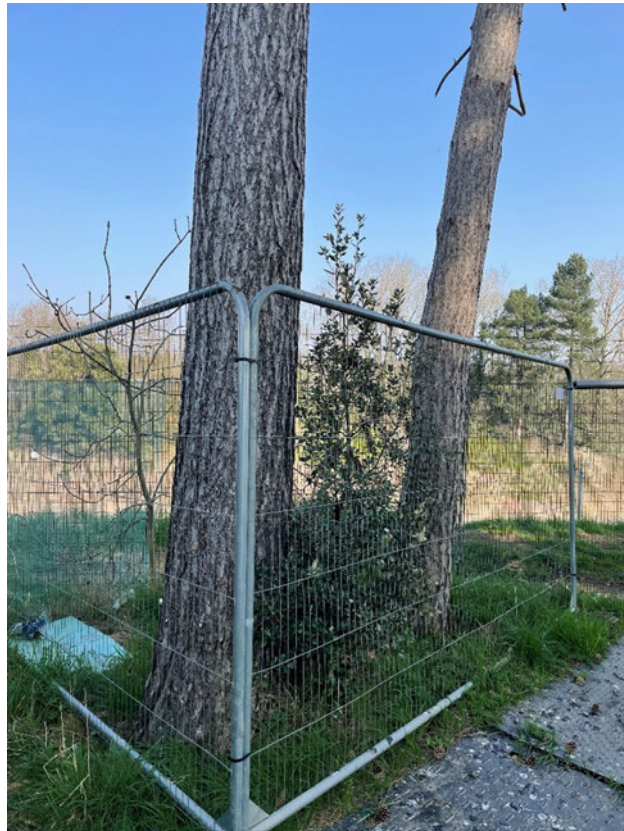
Photo 4; Base of trees 13 and 14, enclosed within Herras fencing.
